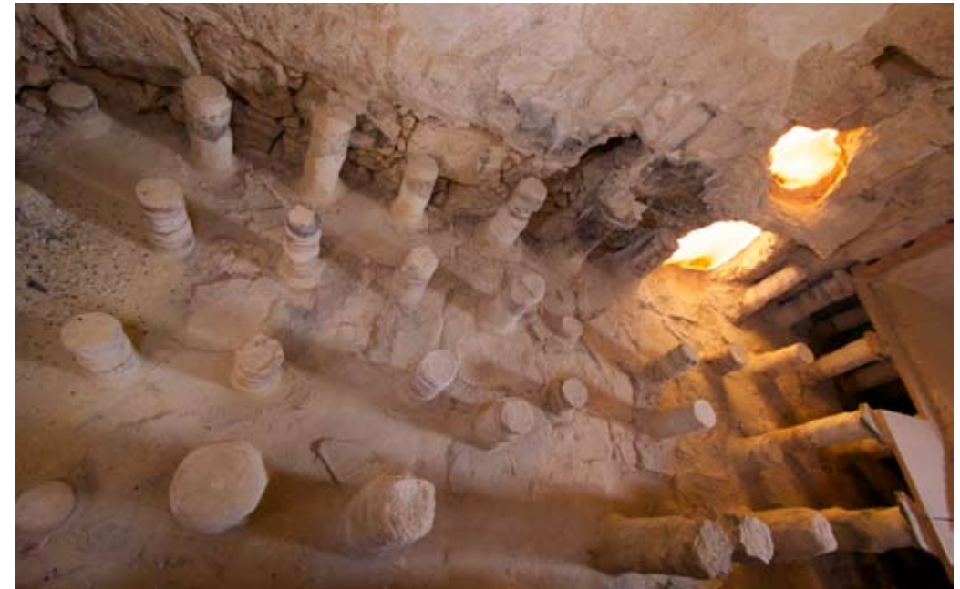
The Calidarium, where hot air circulated beneath a raised floor to heat the room above.
